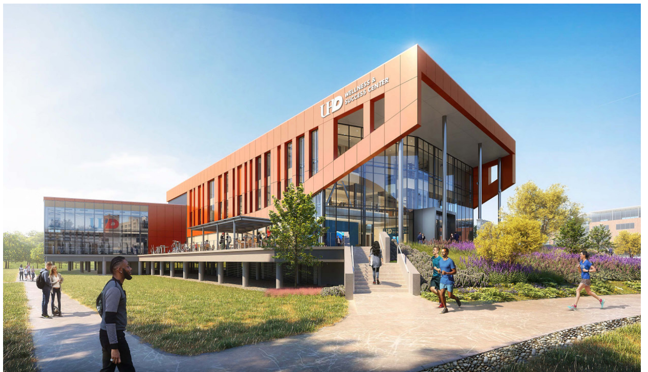
Computer Generated renders of the outside of the future Wellness Center. Courtesy UHD
