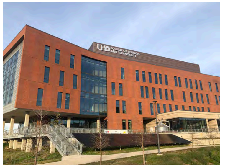
Sciences and Technology Building displays 75 solar panels which power two labs on the first floor of the STB on Jan. 27, 2020. Photo credit: Indira Zaldivar.
