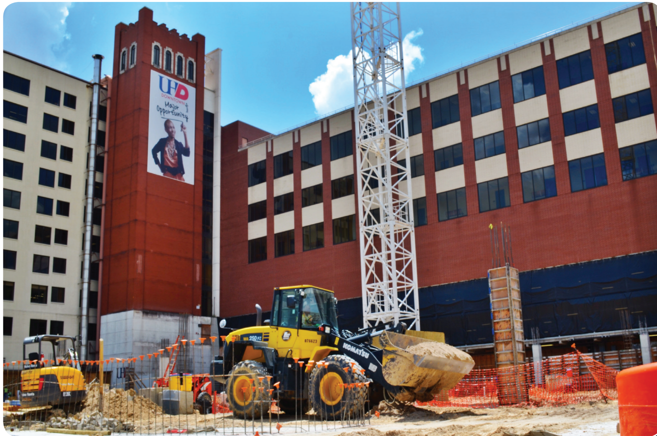
Construction site photos at Academic Building - One Main Street August 8, 2014
