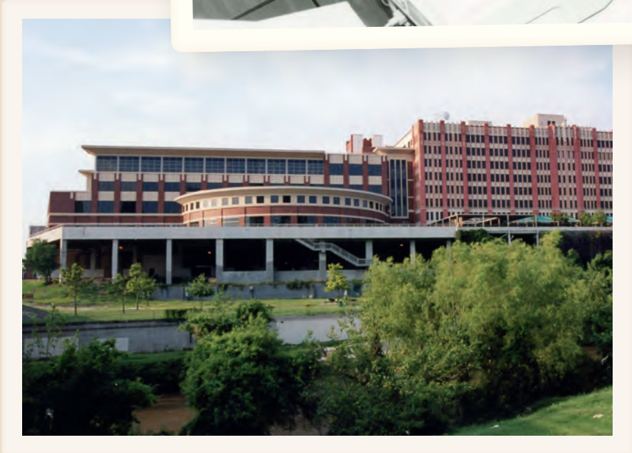
PREVIOUS PAGES: Construction of the Academic Building.
