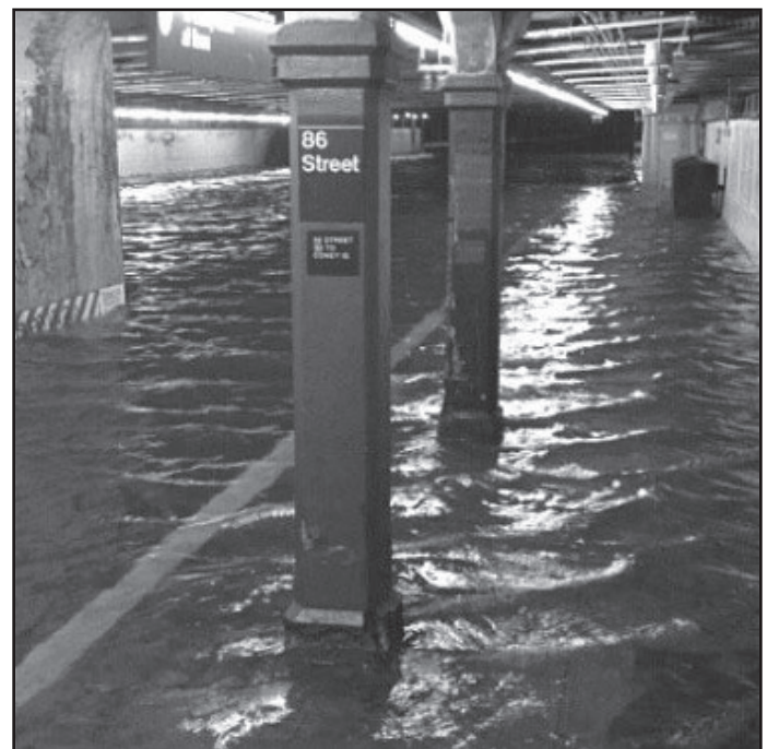
Subway flooding at 86th Street, New York City
